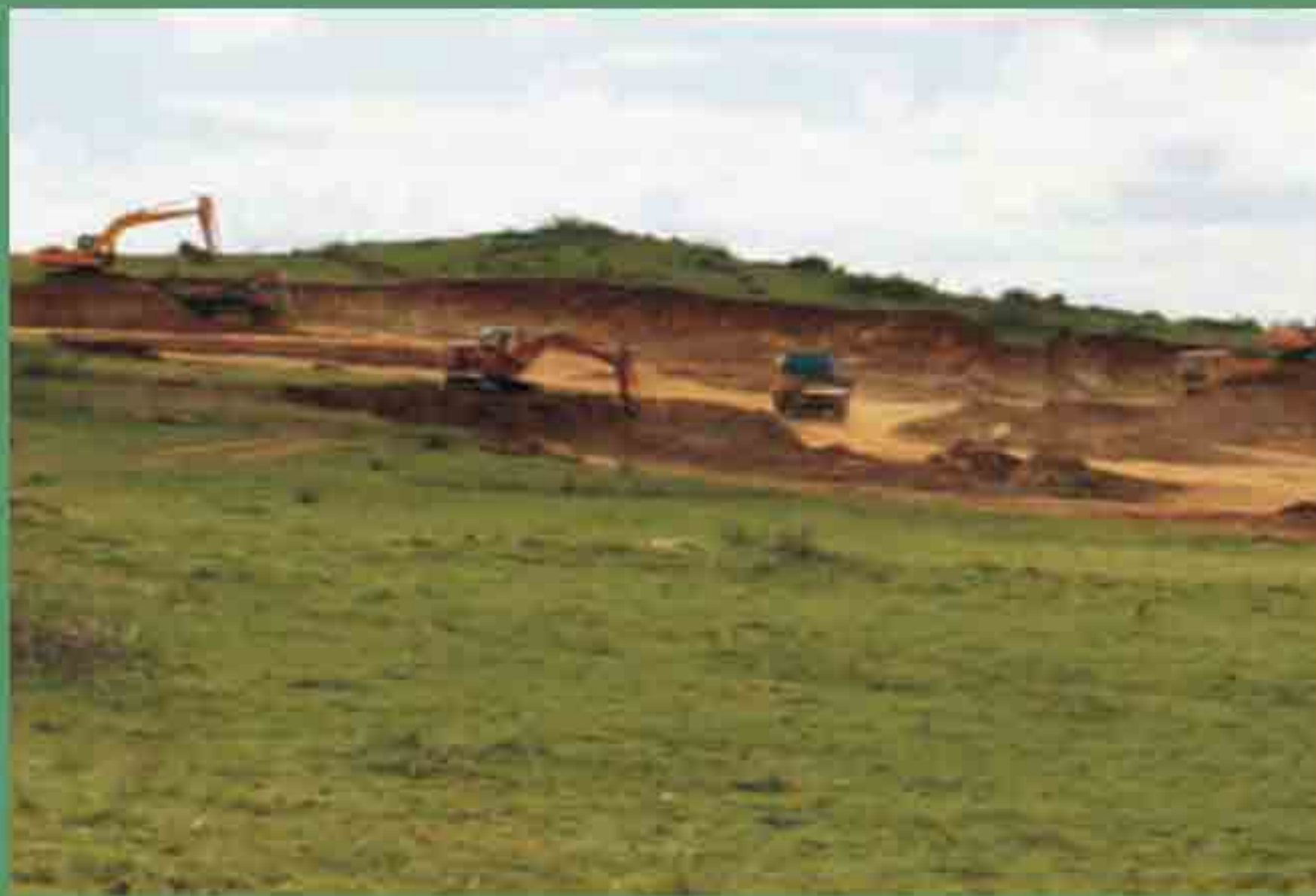
Base Batteries Construction Progress
